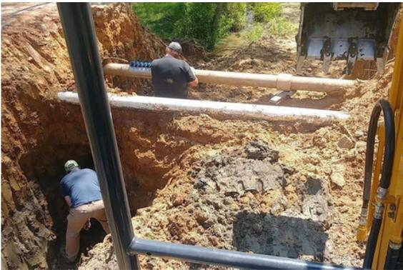
By now you have hopefully noticed a few projects the maintenance staff has been able to tackle this year. **Old rotten drainage pipes are replaced in the ponds on 13 and 18.** A new emergency spillway was constructed on 18 as well. To help with handicaps, a new tee box on # 3 has been built. Finally, the fairway bunker on the right side of #4 fairway was filled in and graded to look like nothing was ever there.
